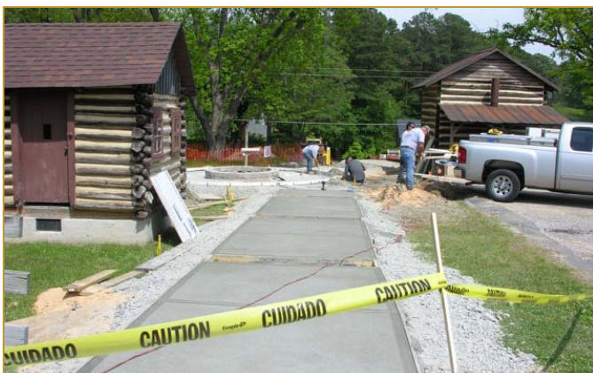
Work underway by playhouse
