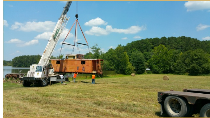
Crane works to move the caboose
